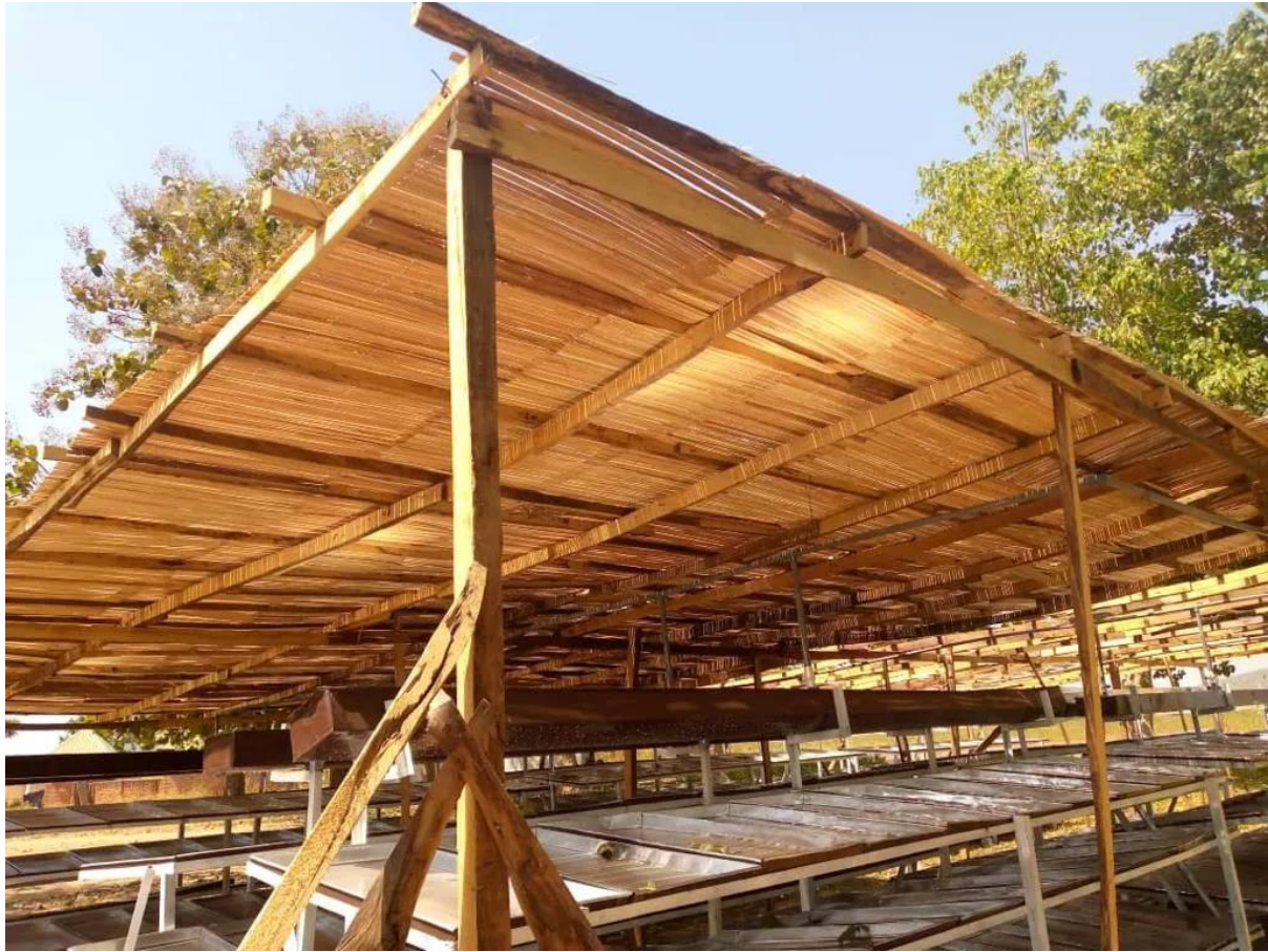
Picture 1: Locally-sourced bamboo roofing materials were trialled as part of the pilot. Photo credit: Bayo Imam
